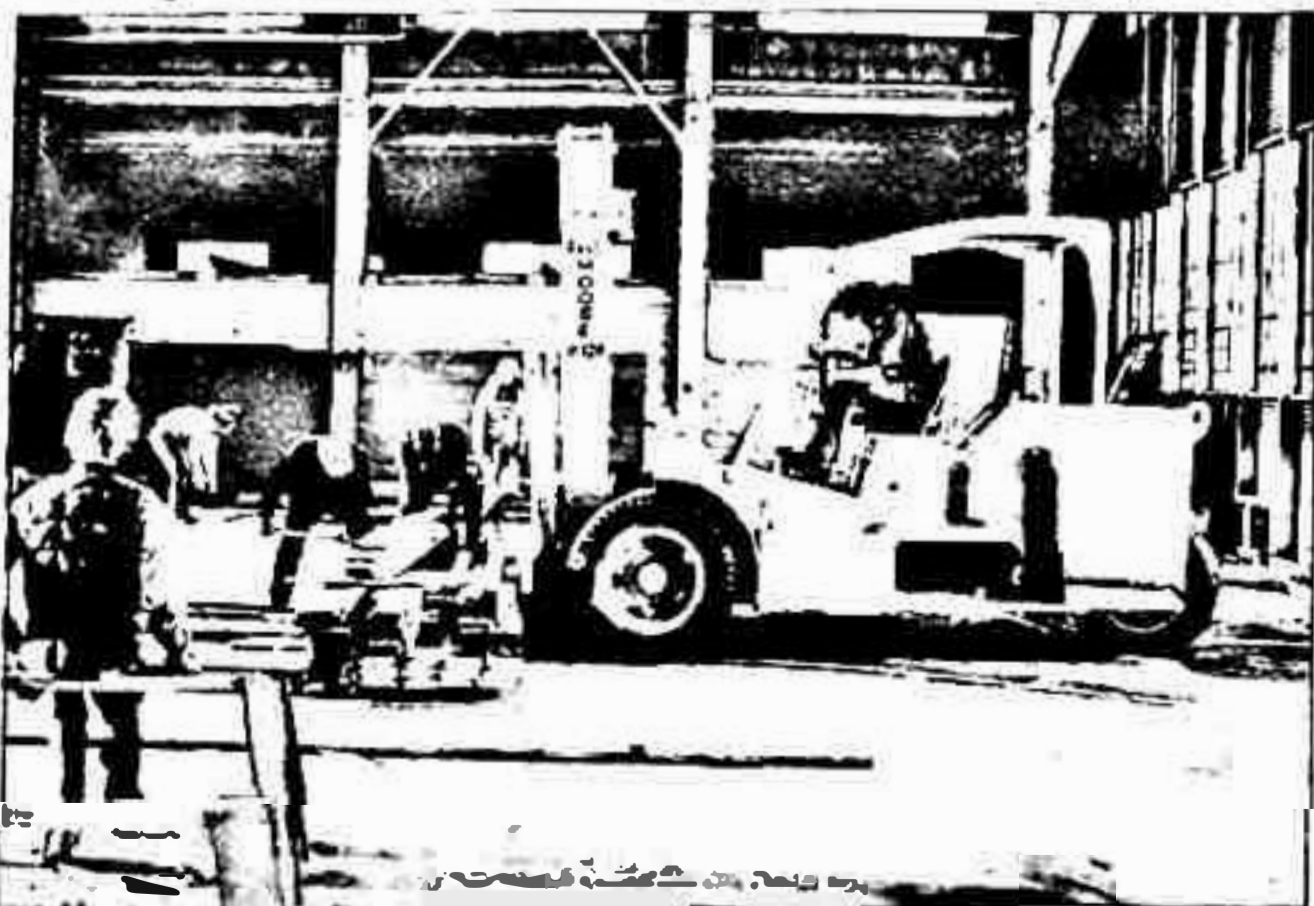
One of five former aircraft hangers at Jericho Beach being used through winter as prefabricating shop for exhibition panels, auditorium seating, etc.
