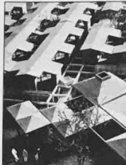
Section of model by second-prize winners Takagi Design Associates of Tokyo, demonstrating use of colonnade as a basic prefabricated structure containing all services. Colonades would be first stage in building, and government-subsidized foundation for inhabitants' self-help.
