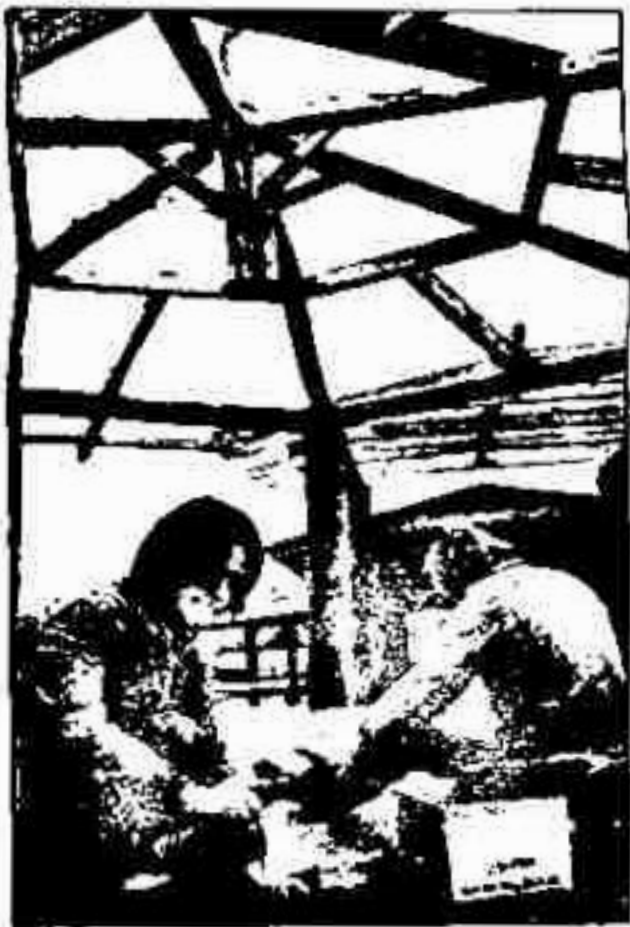
Young workers put down floor on covered walkway leading into large Forum complex. Logs are driftwood picked up at local beaches covering roof consists of discarded corrugated sheeting — but the rafters are new.
