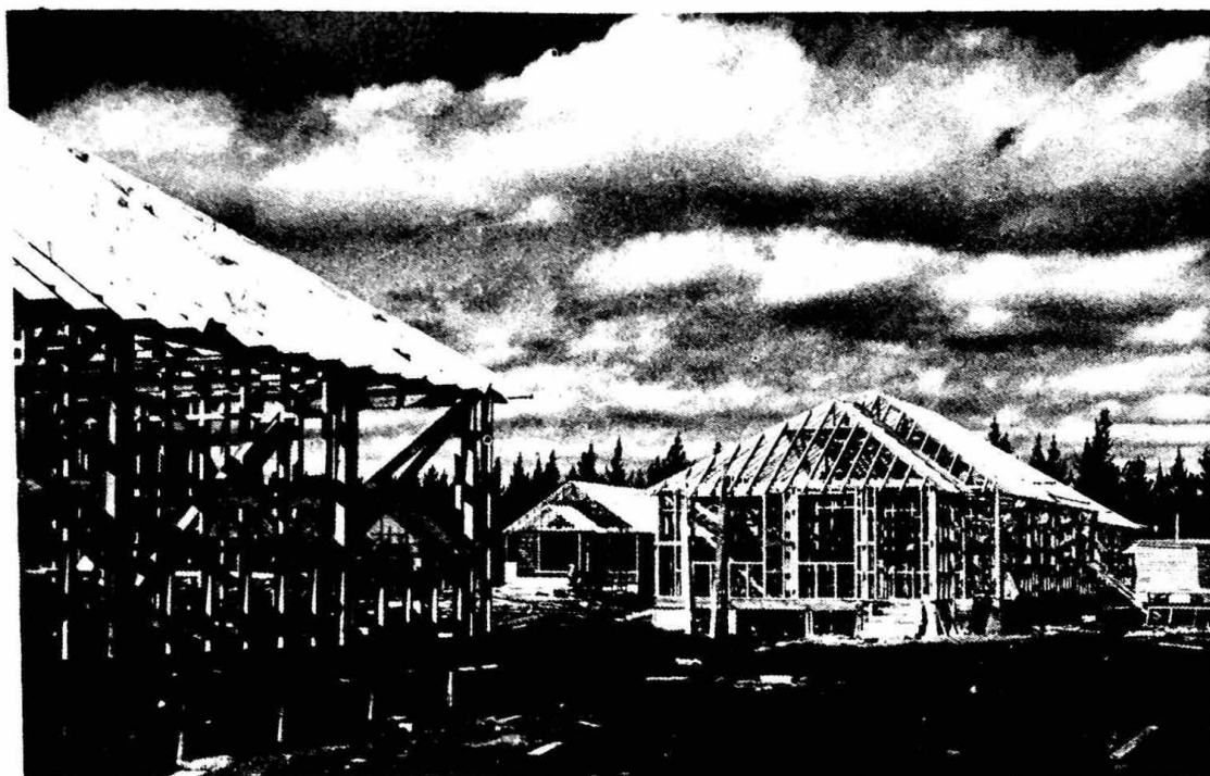
Houses almost entirely of radiata pine, including the sub-flooring, which is of treated timber.
