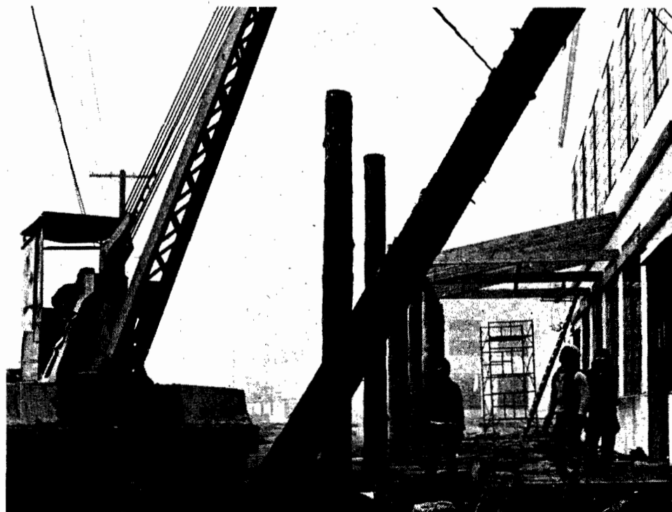
LOG RAISED... walkway under construction
