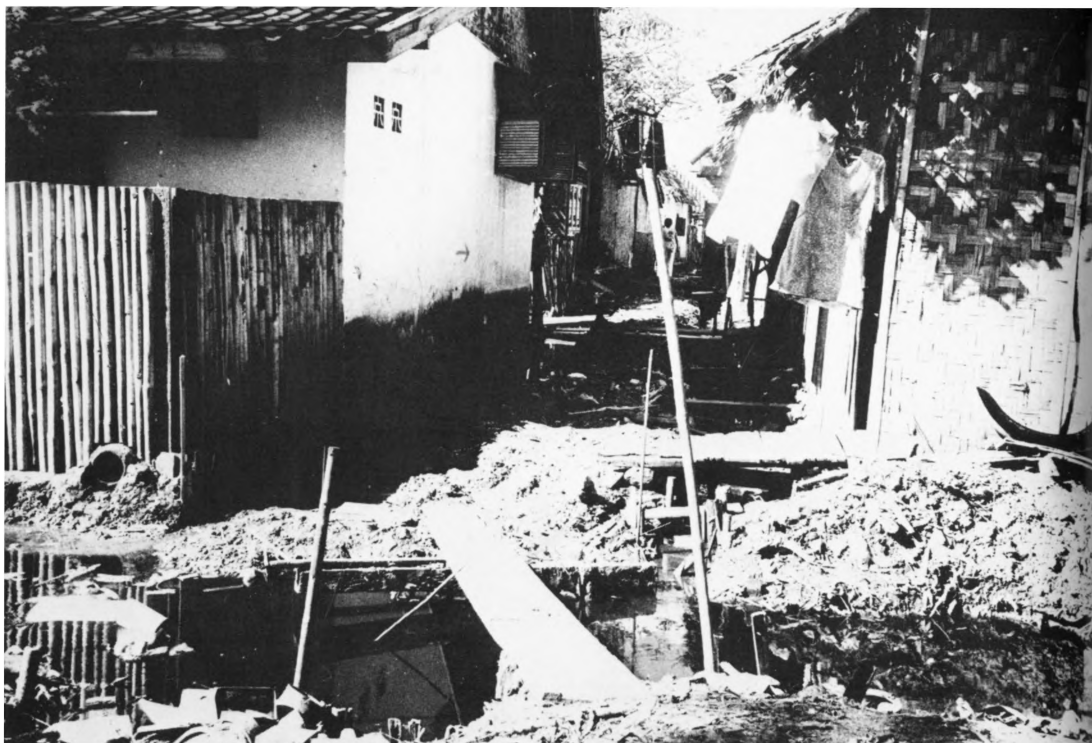
6. Some hope and promise — Kampung Improvement Programme in Jakarta, started in 1975.
